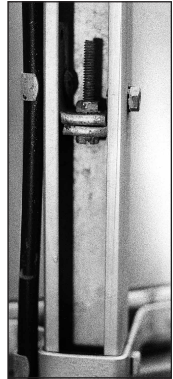
Fig 13—In this photo the open edges of the Unistrut channel are facing the viewer. The locking pin is visible in the middle of the channel.
